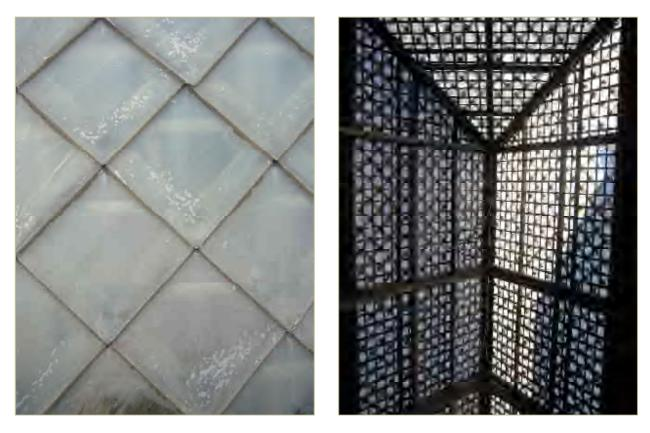
Figure 19. Left, detail of the glass slates from above. Right, the effect of the glazed roof from below
