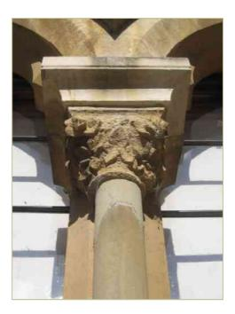
Figure 13. Damage to capital on southern tower of western elevation
