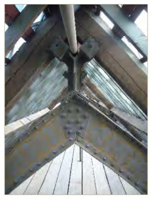
Figure 11. Rafters, trusses, and brackets within the roof space
