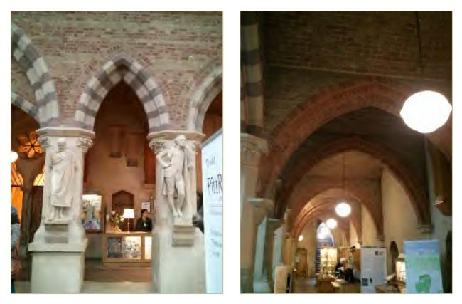
Figure 20. Left, brickwork and banded stone arches on the western end of the central court. Right, barrel vaulting along the ambulatory at the western end of the central court
