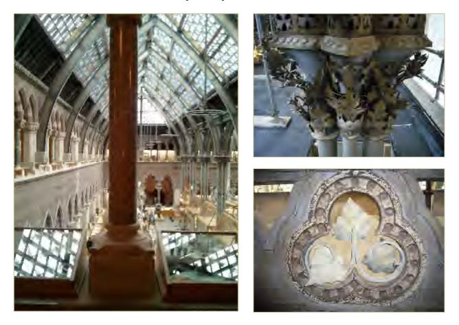
Figure 18. Left, iron columns and arches in the northernmost aisle of the central court. Top right, wrought iron floral decoration on pillar capitals. Bottom right, wrought iron floral decoration on horizontal truss
