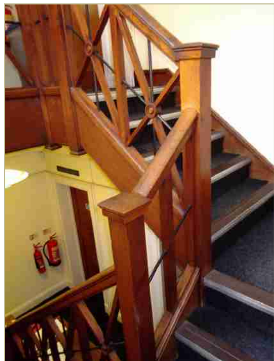
Figure 11. Joinery on the staircase in the 1925 extension
