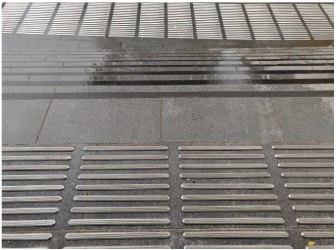
Aluminium corduroy strips are a slip hazard when wet and should be avoided
