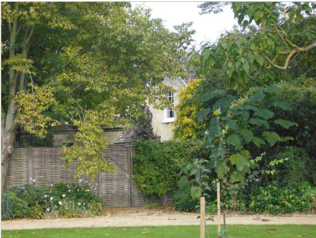
Figure 12. The upper storey of the Grade-II-listed Cottage rising above the surrounding fence and foliage
