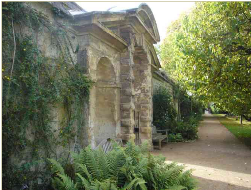
Figure 10. The eastern gateway and wall looking southwards
