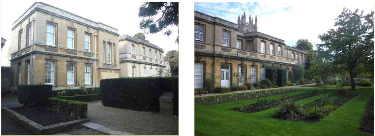
Figure 21. Left, the West Block from the north looking southwest. Right, the West Block from the south, looking northeast
