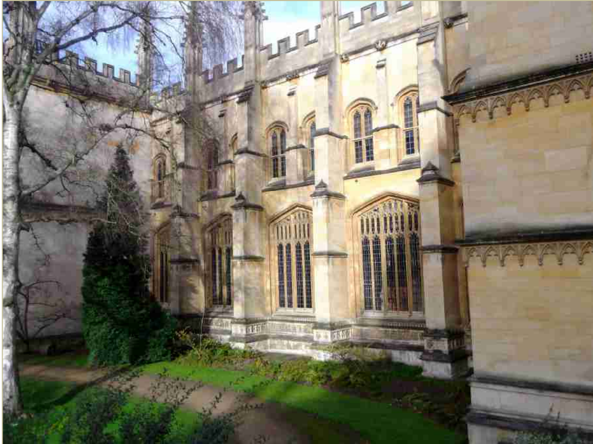
Figure 18. The southern elevation of the Divinity School and Duke Humfrey's Library
