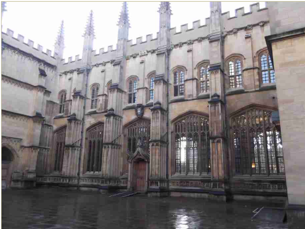
Figure 17. The northern elevation of Duke Humfrey's Library and the Divinity School without highlighting. Note Fisher's 1669 doorway in the central bay
