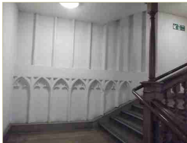
Figure 31. 31.1. Top left, the 2011 internal lobby to the ground floor of the northeast stair tower. 31.2. Top right, the staircase in the north-western stair tower looking north-eastwards. 31.3. Bottom, the obscured panelling of Arts End preserved in the western wall of the north-western stair tower
