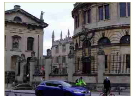
Figure 13. 13.1. Top, the view southwards down Catte Street. 13.2. Middle, the northern elevation of the northern range of the Old Schools Quadrangle. 13.3. Bottom, a glimpse of the Old Bodleian between the Sheldonian Theatre and the Clarendon Building looking southwards
