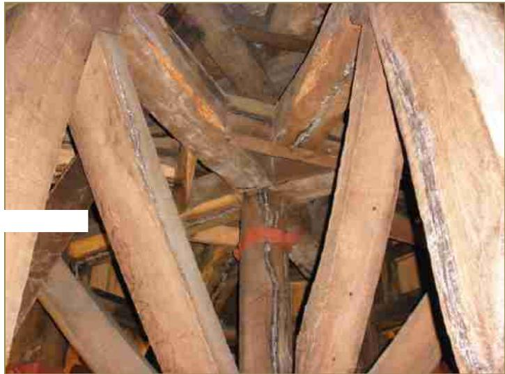
**Figure 7. The complex timber construction of the interior of the dome**
