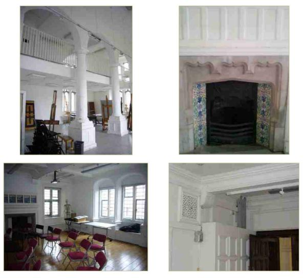
Figure 13. 1. Top left, first-floor double-height space with mezzanine. 2. Top right, original fireplace in second-floor room. 3. Bottom left, first-floor room ('Censor's Room') with original fireplace. 4. Bottom right, electrical trunking etc. in first-floor room
