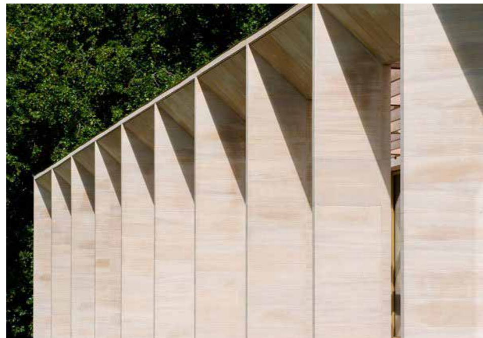
Clipsham stone used for stone pillars at Sultan Nazrin Shah Centre, Worcester College
