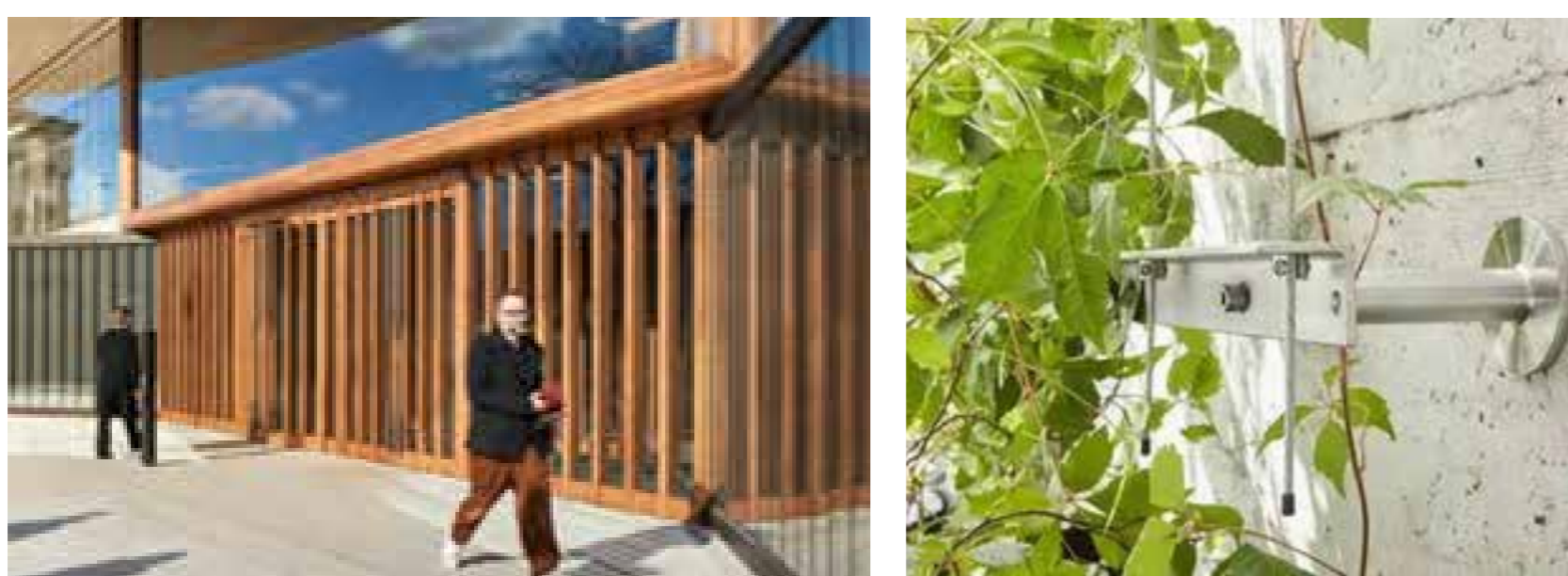
Top: Reflective glass used at St Antony's College and the Blavatnik School of Government. Bottom: Use of timber screening at Blavatnik Institute and example of green wall on stone
