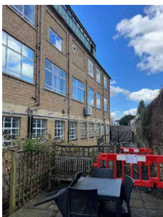
Photos of existing Gibson Building façades
