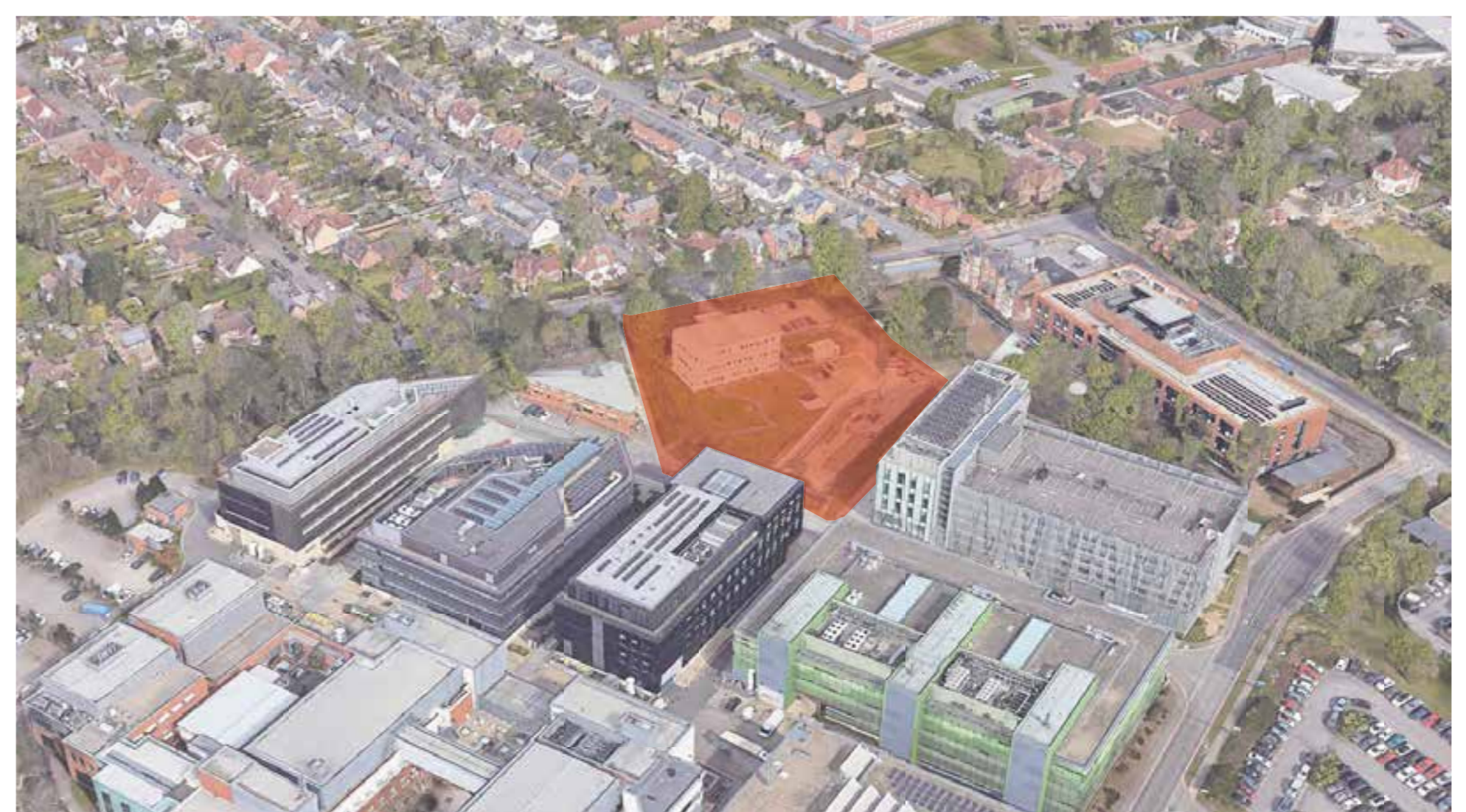
Aerial view showing the Plot B2 site and its location within the Old Road campus
