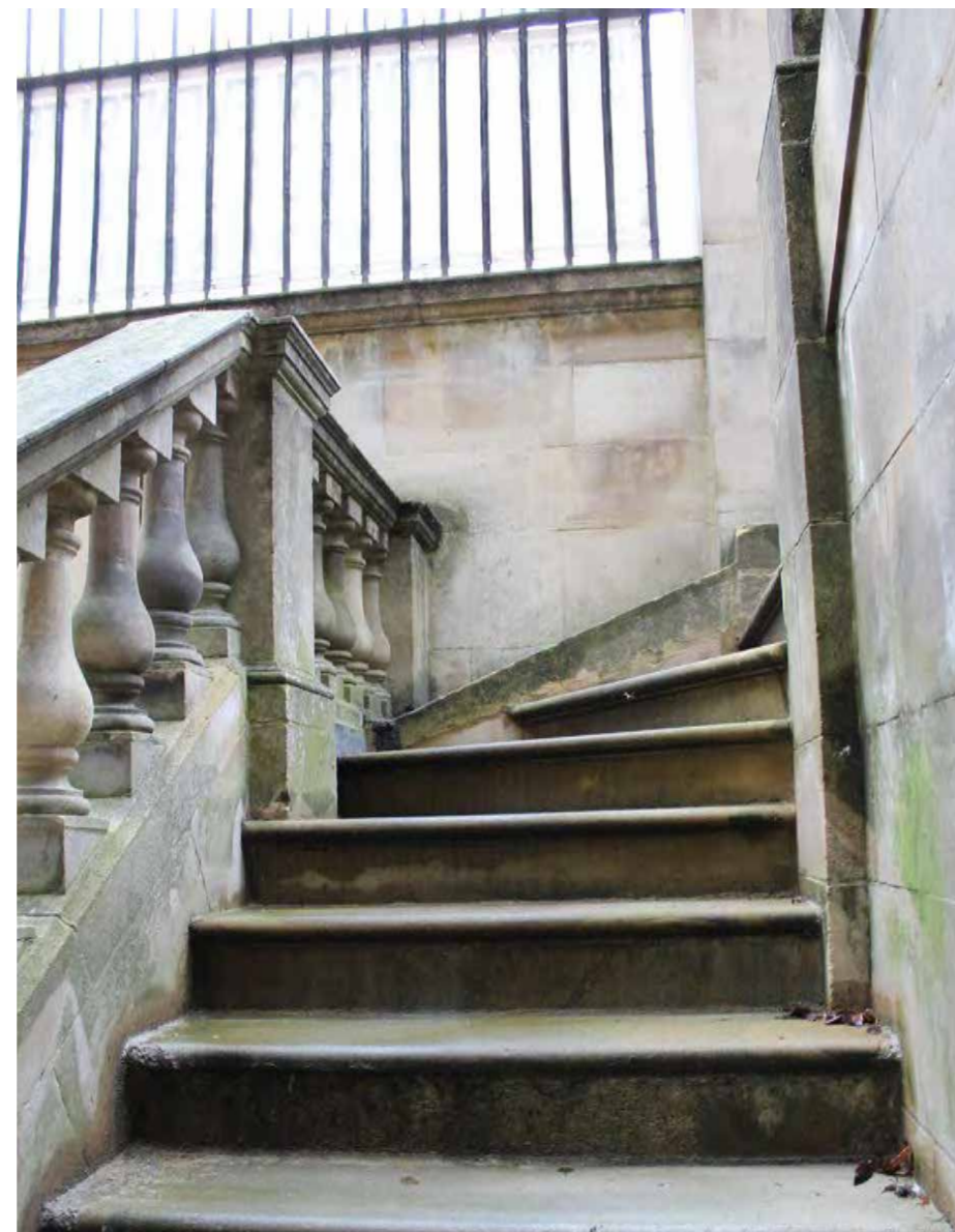
Existing external staircase
