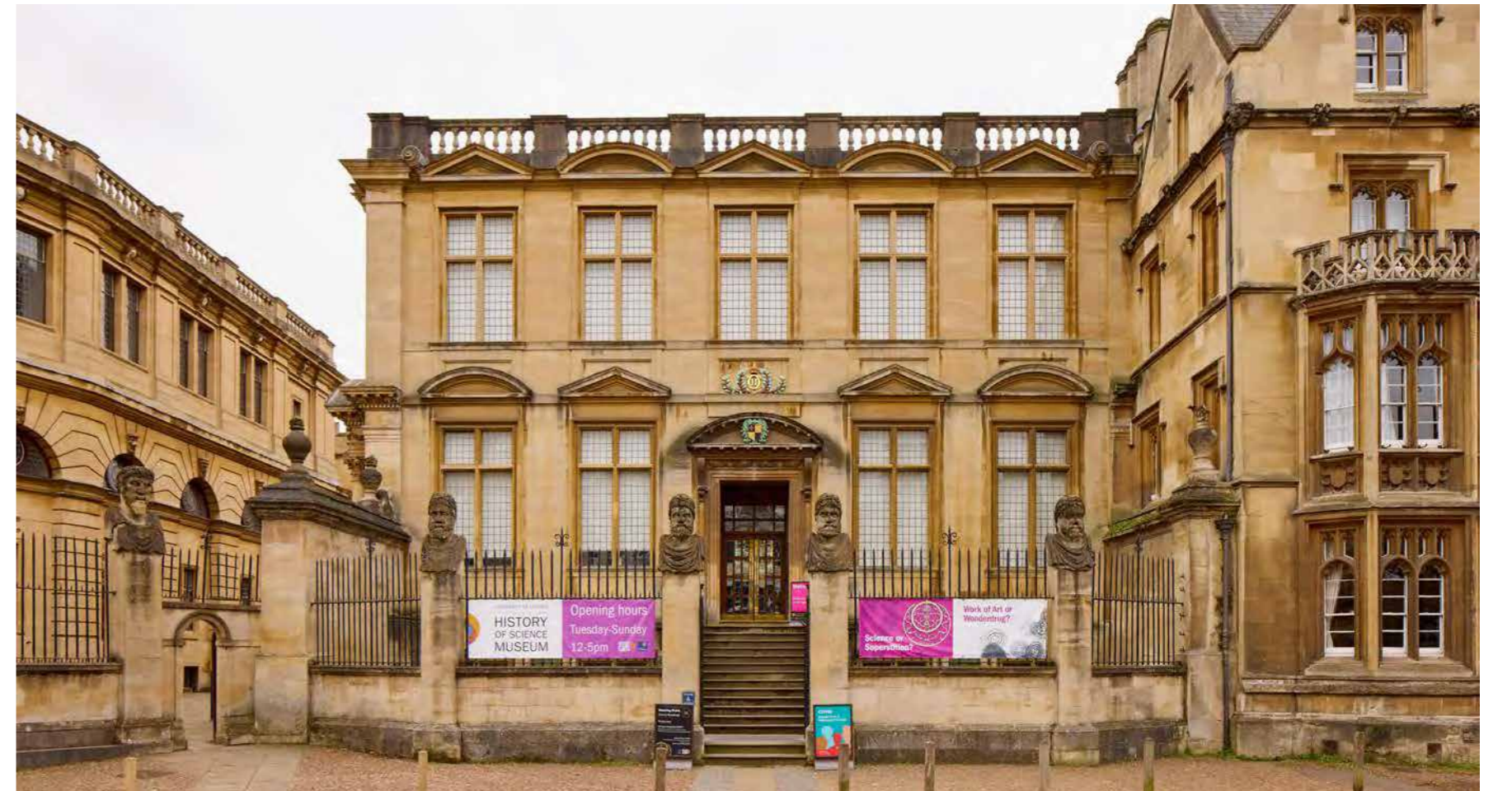
Existing access via a steep flight of stairs
