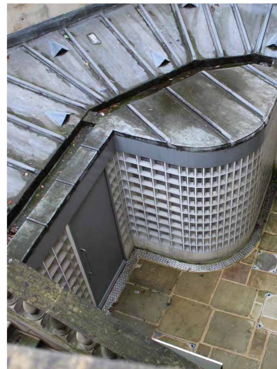
Existing basement extension roof
