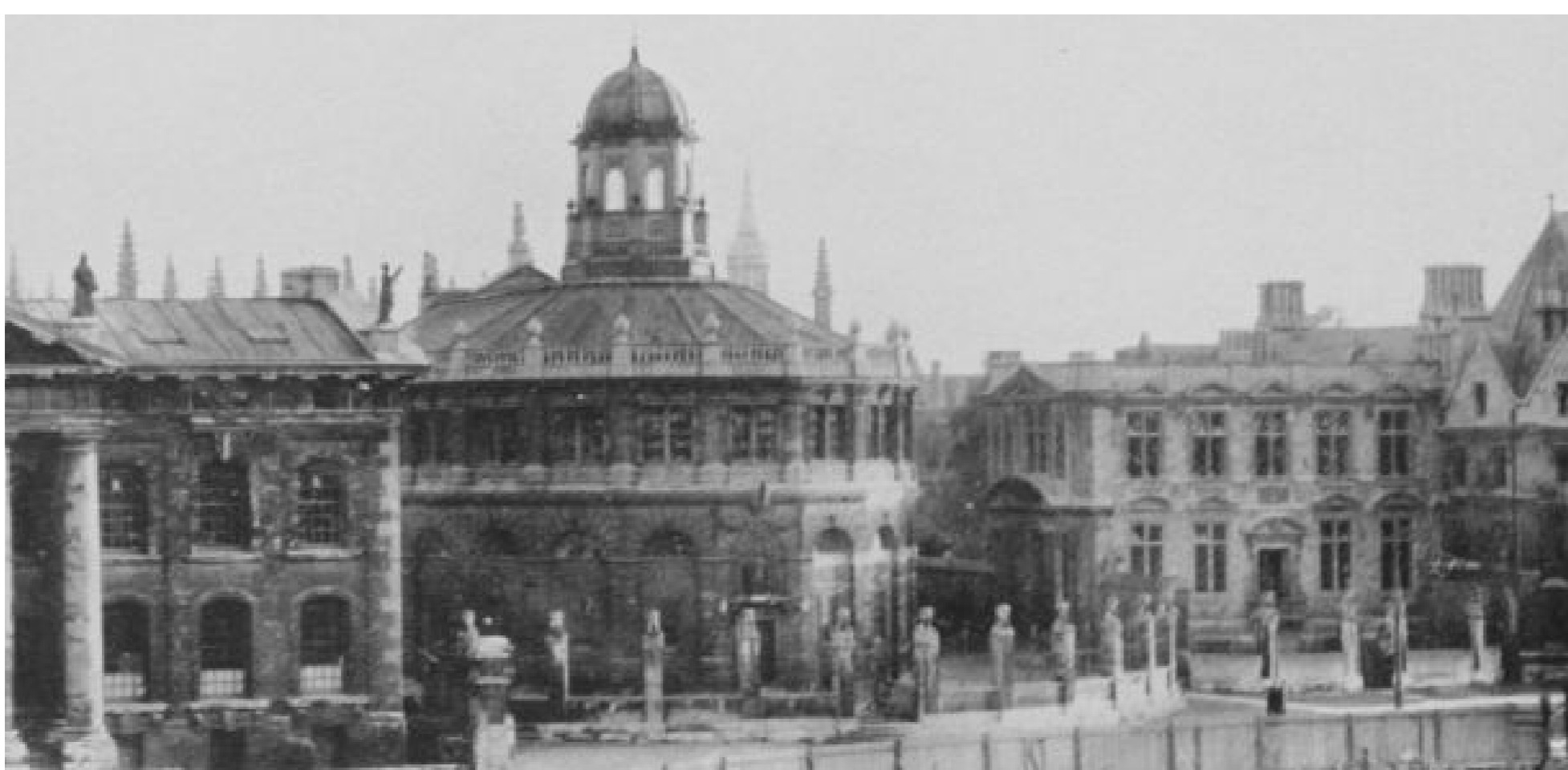
View of Broad Street, 1939
