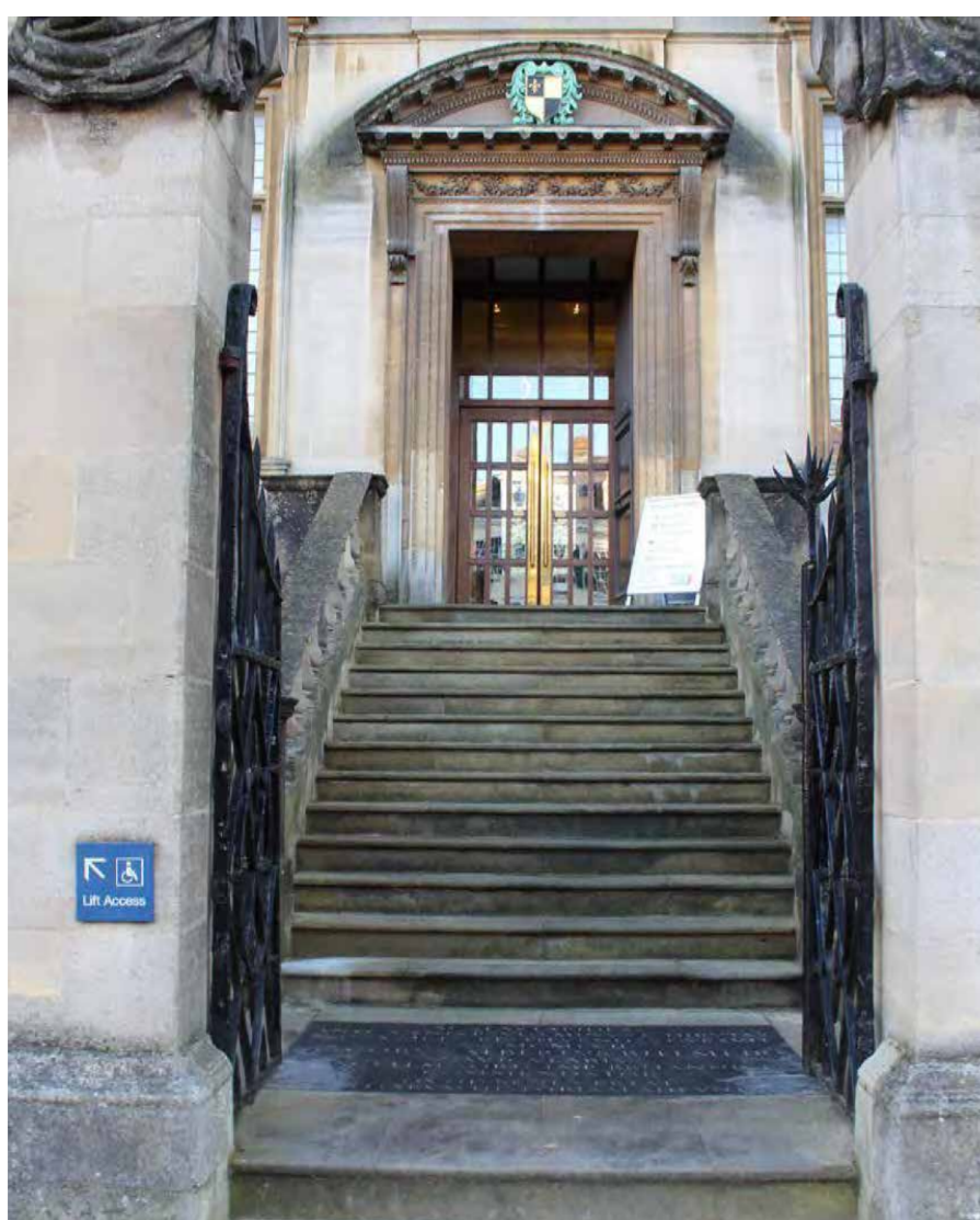
Existing Broad Street steps
